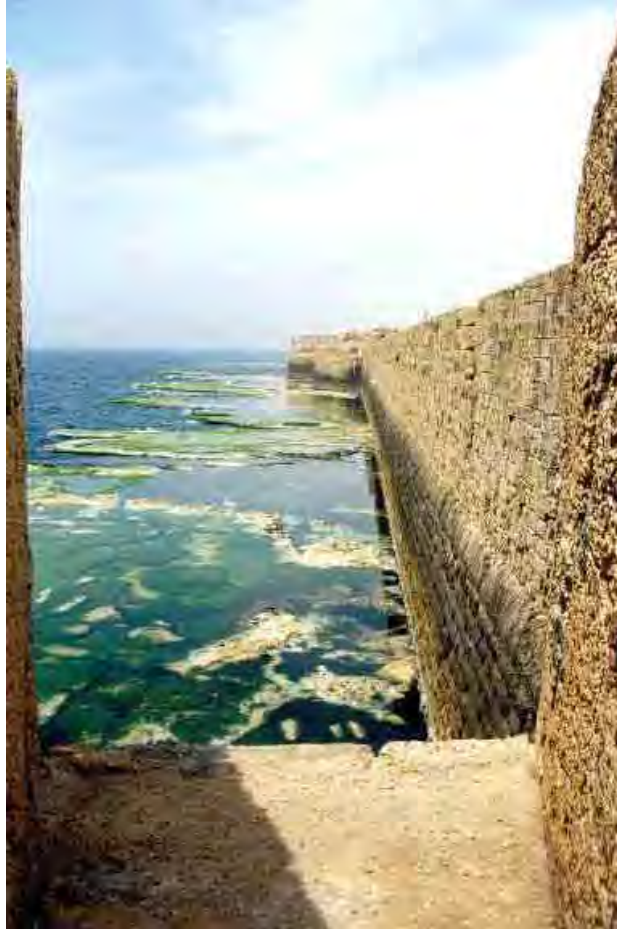
Sea wall at Acco
